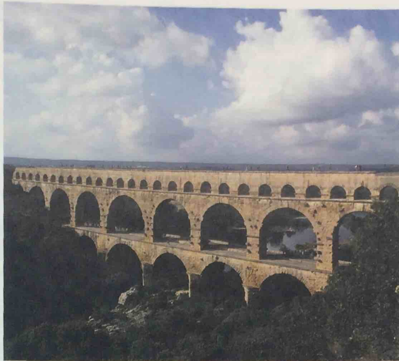
>> The Pont du Gard in France was a Roman aqueduct built in 19 B.C. The three tiers of arches rise about 155 feet (47 m).
